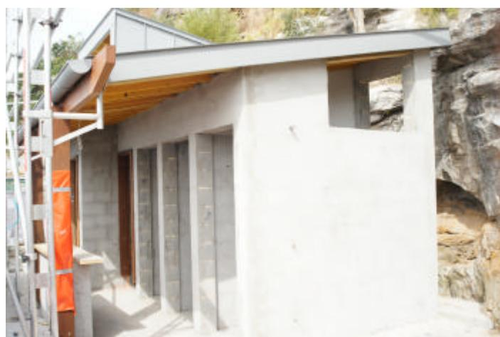
**The reconstruction of the Fairy Bower Pool Amenities block continues.** Here progress up to 6th of October is shown. The basic building structure including the roof is now complete. The door and window installation has commenced, with ceramic tiling also about to start.
