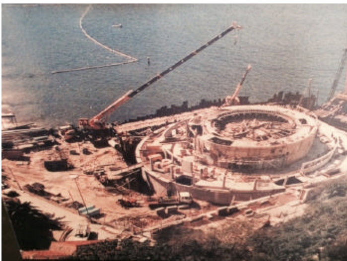
Manly Underwater World under construction in late 1987. This photo particularly shows the sheer scale of the aquarium structure - note the new tunnel walk compared to the original tank size. (image Manly Sea Life Sanctuary)
