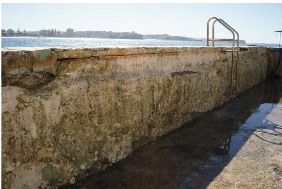
The end wall of the pool showing the limited water depth with little capacity for any reduction, and the edge topping coming loose and needing replacement.
